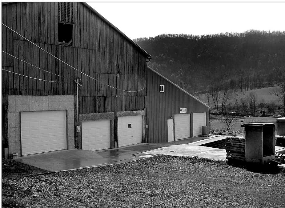
Appalachian Harvest began operations in a tobacco barn in Stickleyville, VA to which modifications and additions were added over several years.
